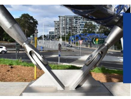
LACHLANS BRIDGE is an award winning pedestrian and cycle bridge in SYDNEY, AUSTRALIA. Completed in 2020 and designed by ARUP AUSTRALIA this unique helix shaped bridge features M76 and M90 Duplex stainless compression struts with special Inconel 718 pins and spherical bearings to meet potential misalignment in the structure.
